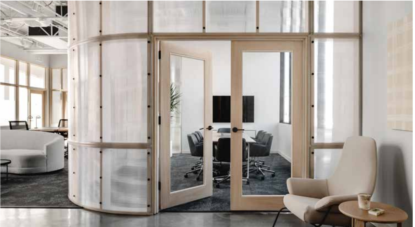
CONFERENCE | Shared conference room directly at entry, light filters through translucent polygal construction
